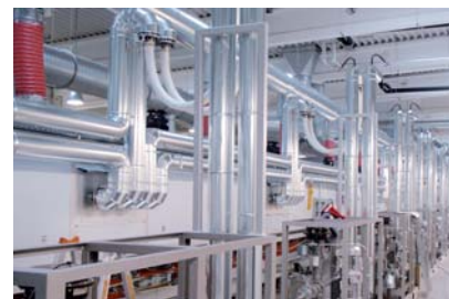
Drive side of dryer
